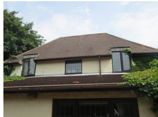
Existing rear roof view.
